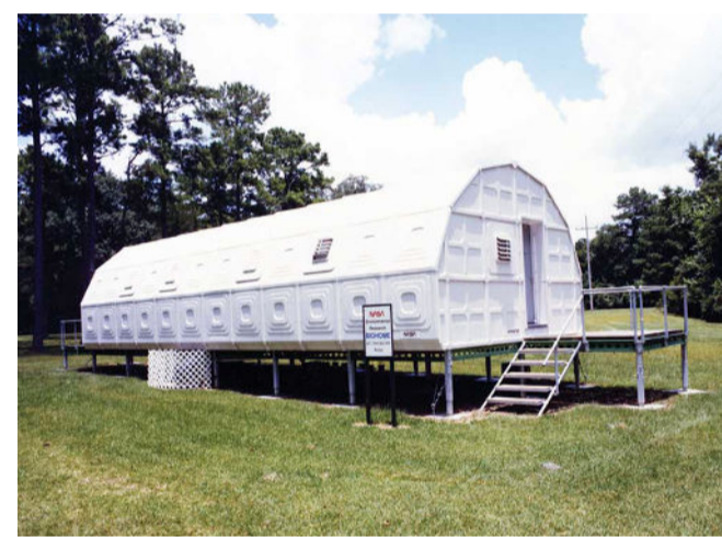
The BioHome at NASA's Stennis Space Center was 45 feet long, 16 feet wide, and used common indoor house plants as living air purifiers.
